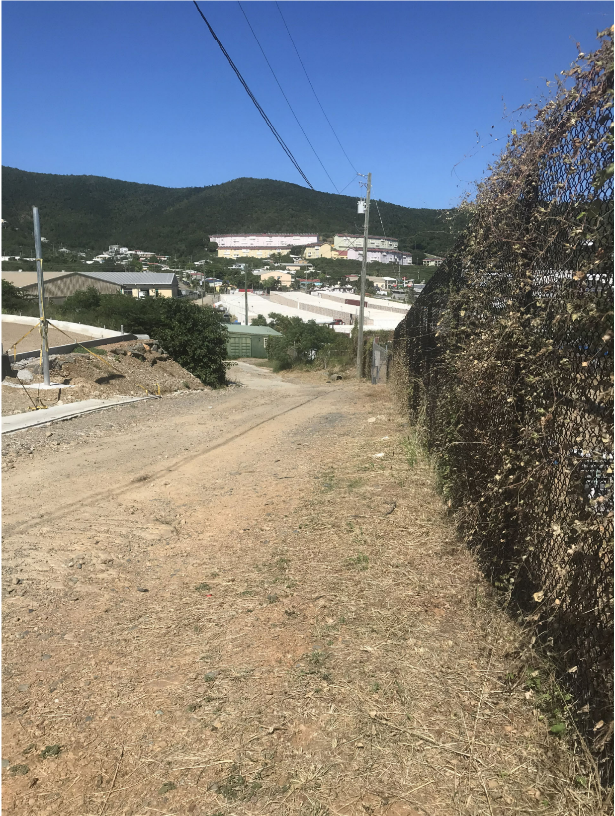
Looking north down Trailer Road from southwest corner
